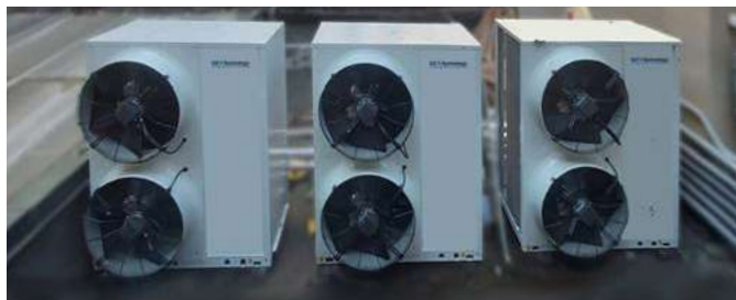
Starting from the left, 437.27 kWp photovoltaic system, 180 kWp photovoltaic system, 3 BWHE281 air-water heat pumps in cascade.
