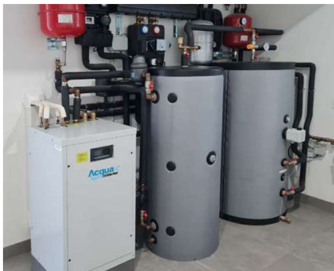
System with Acquainverter® heat pump model WM15 with 2 external units completed with a 200 liter WACN thermal flywheel for chilled and heating water and a 300 liter WBX domestic hot water thermal storage tank integrated with the solar thermal system. The system was integrated with 8.68 kWp solar photovoltaic.
